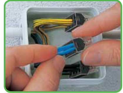
Wire Removal Solid - Pull & Twist; Remove wire Stranded - Cut Wire; Discard connector Restrip conductor and insert into new connector
